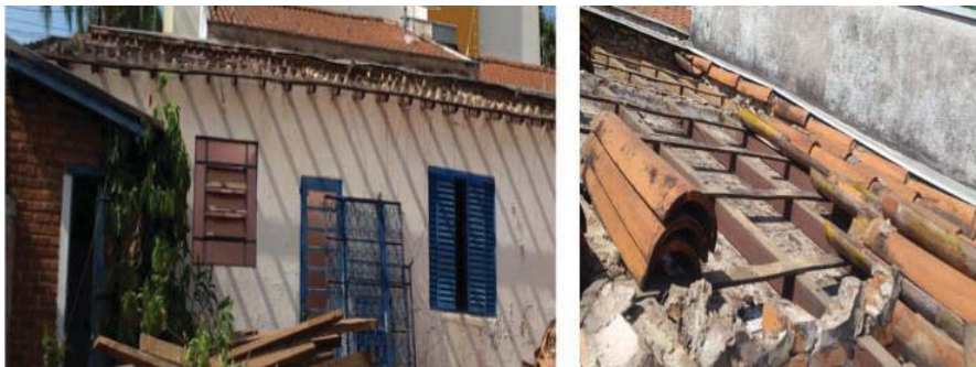
Figure 9 and Figure 10. Removing the coverage of the building. Source: Author, 2015
