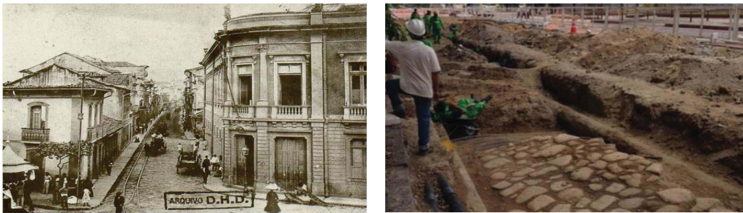
Figure 1. (Left) - Ajuda street at the beginning of the 20 th century with sidewalks in granite stones; (right) - Stone sidewalk in "pé-de-moleque" style on Rio Branco avenue, Rio de Janeiro.
