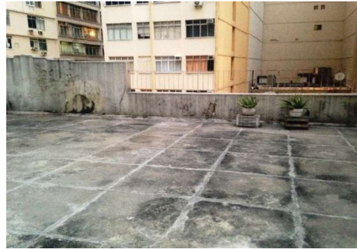
Figure 4: Conventional roof, Source: Author, 2016
