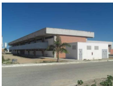
Figure 4. Building of classrooms - Longitudinal northeast facade, 2014
