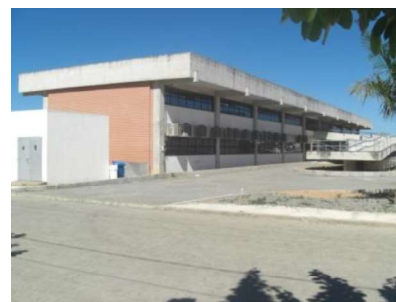
Figure 5. Building of classrooms - Longitudinal southwest facade, 2014
