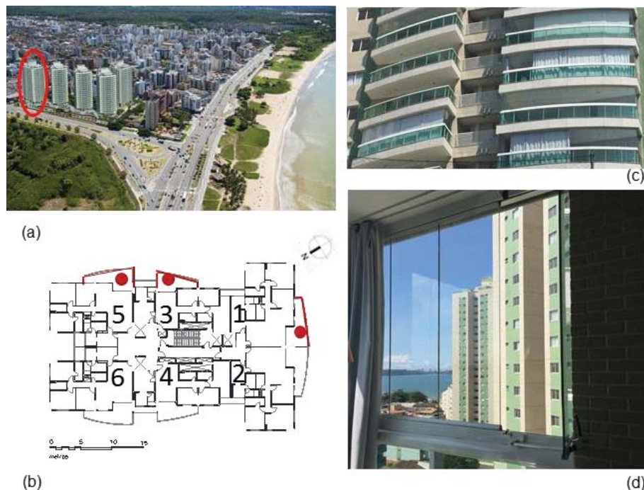
Figure 1. (a) Emphasis on monitored building and (b) the distribution scheme of the apartments with the location of the monitoring points in columns 1, 3 and 5. Emphasis the balconies. Source: adapted from Galwan (2016). (c) balconies in the southeast facade (d) Glazed balcony of 10 th floor.
