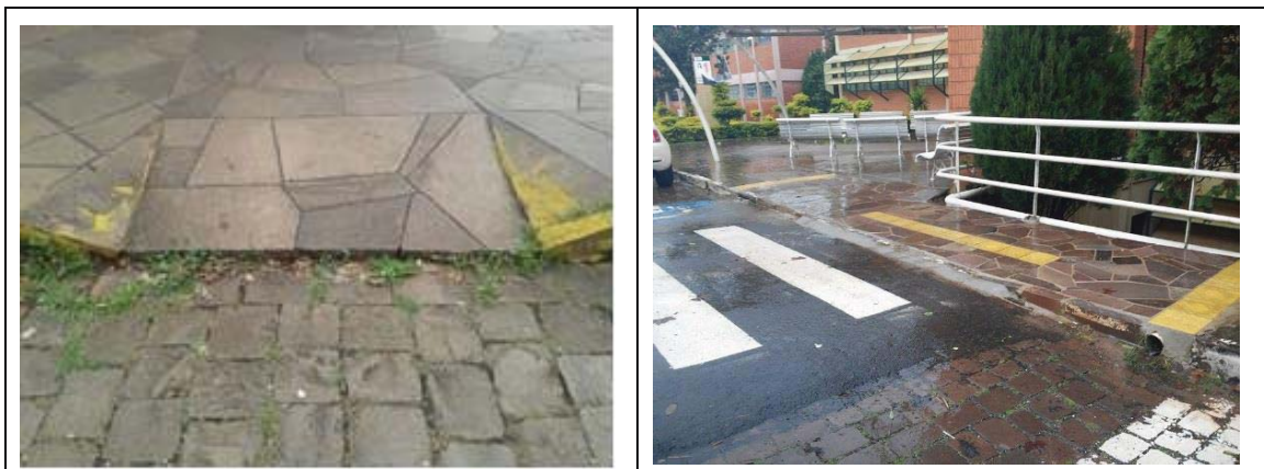
Figure 3. Ramp before and after modifications. Source: Authors, 2015.
