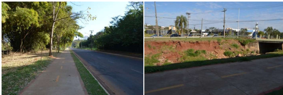
Figure 7. Francisco Pereira Lopes Avenue highlighting the bike path and landslide of the slope (photo on the right)
