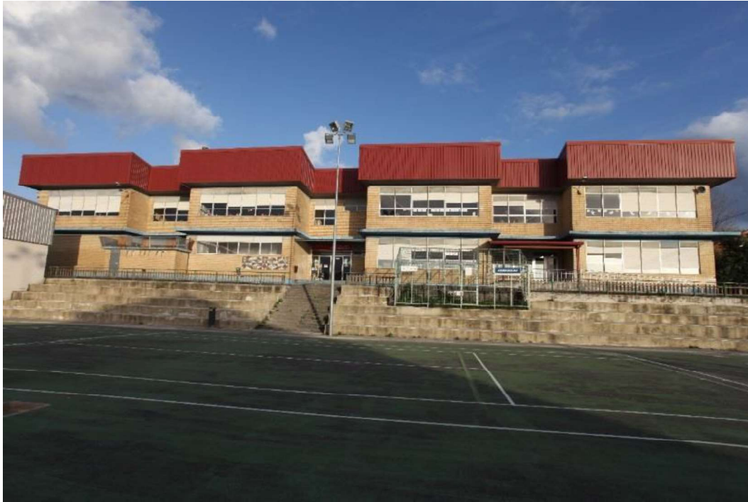
Figure 1. Study case. San Roque Elementary school in Cangas, Pontevedra, Galicia, España. West facade.
