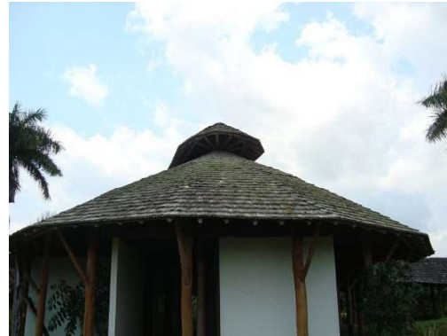
Photos 7 and 8 - Zenith openings in the main cover
