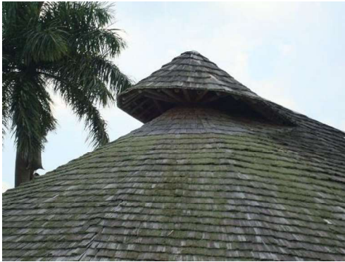
Photos 7 and 8 - Zenith openings in the main cover
