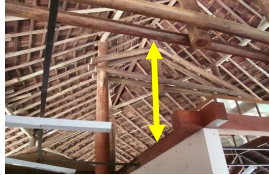
Photo 6 - the roof reaches a height up to 8 meters creating an air protection
