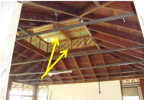
Photo 9 – Double protection and zenith ventilation
