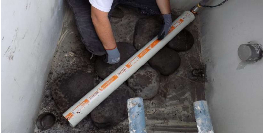
Figure 2. Installation of the submersible pump
