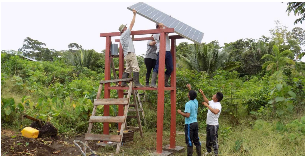
Figure 3. PV panel installation
