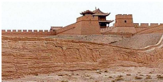
Figure 1. Great Wall of China. Some sections Built of rammed earth. Construction began around 220 B
