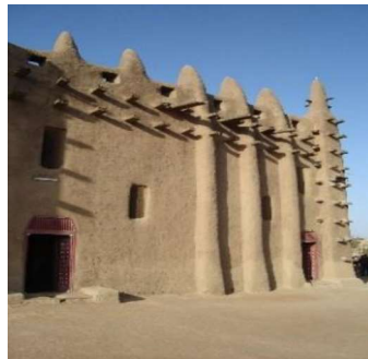
Figure 6. Djenné Mesquite, Mali. The largest building made of earth with its original use today (1240 AJ)
