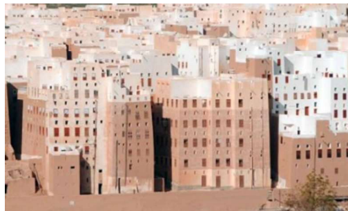
Figure 2. View of the City of Shibam Yemen. Multi-story natural earth high rise buildings 500 year old. The oldest skyscraper in the world. UNESCO World Heritage from 1982
